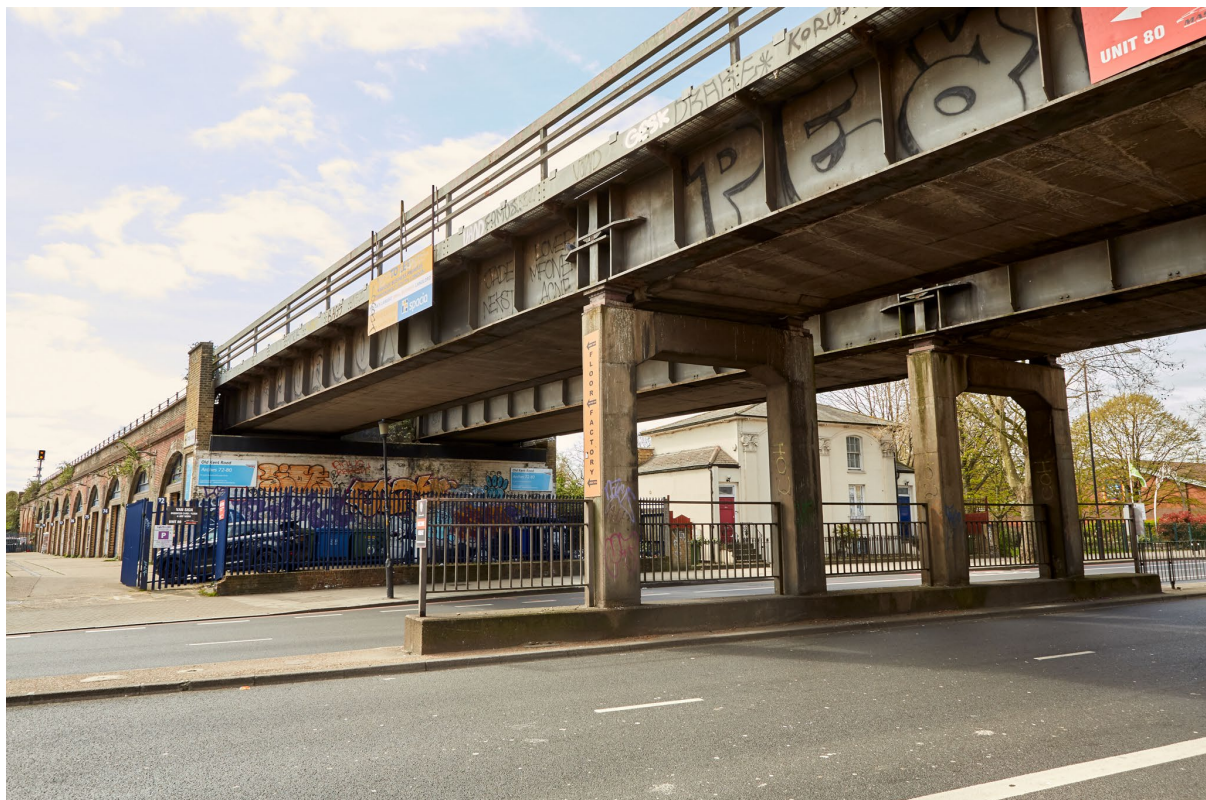
Railway Bridge from New Cross side looking towards Southwark side
