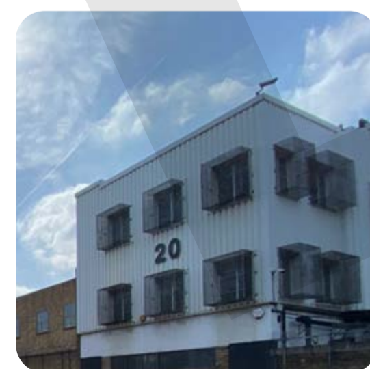
Protruded elements and structures, breaking the plain elevations.
