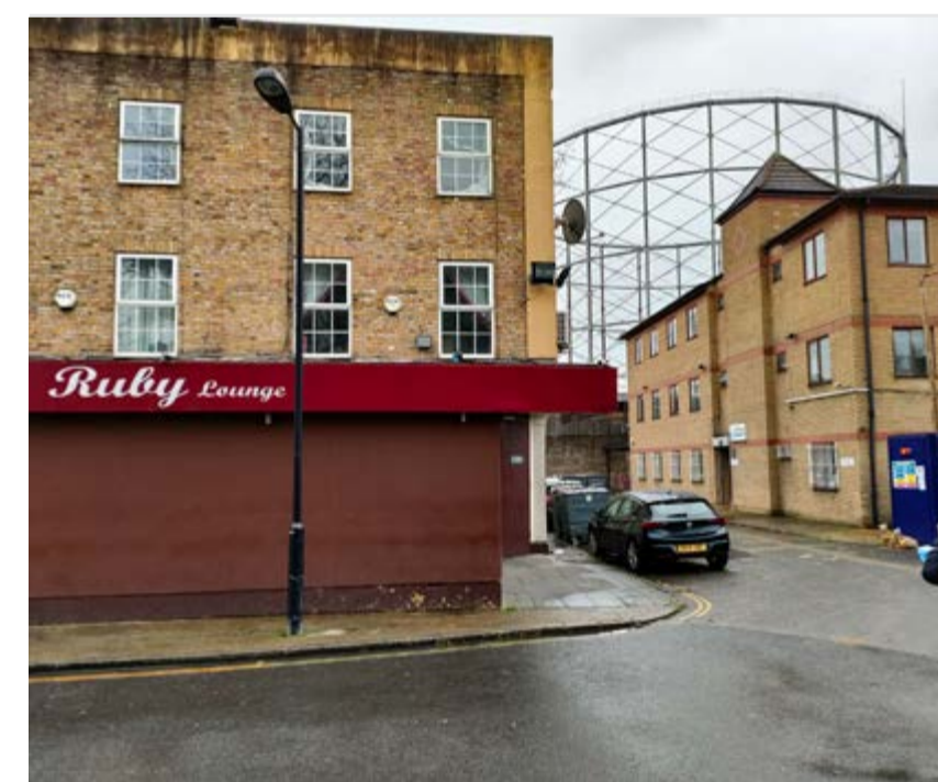
Scale and contrast of traditional buildings and structures (Gasholder)
