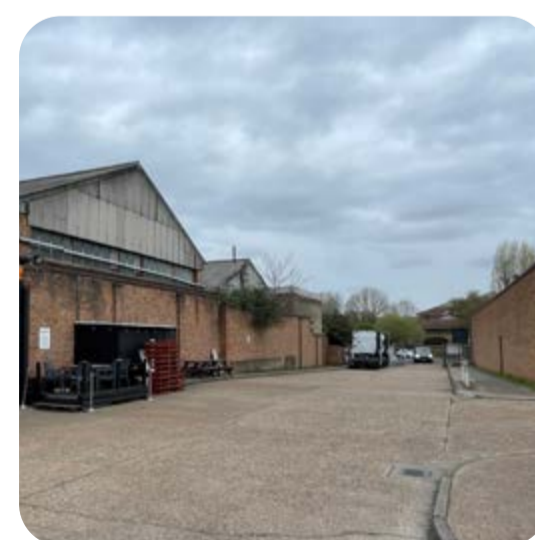
Brick base with top horizontal metal band, plain brick work and pitched roofs speaking to industrial heritage.
