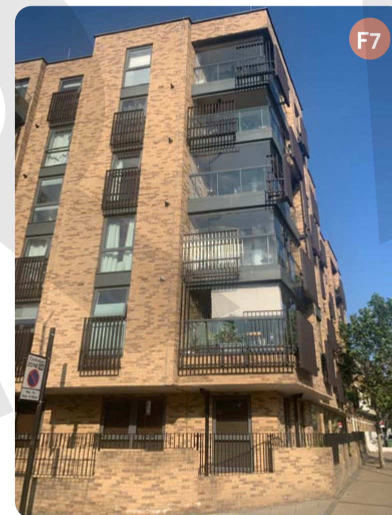
Enclosed balconies (or winter gardens) reduce noise entering a building. Enclosed balconies may require ventilation. Acoustic louvres could also reduce noise and ventilation requirements
