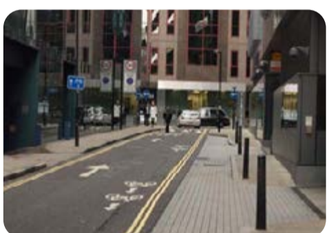
Inset loading facilities
