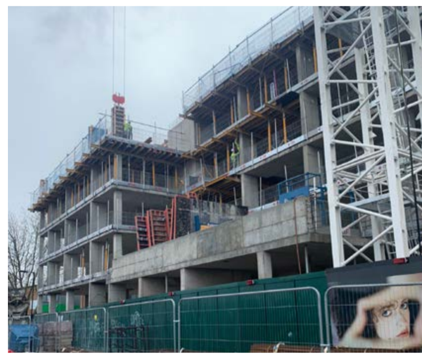
An area of change with multiple construction sites
