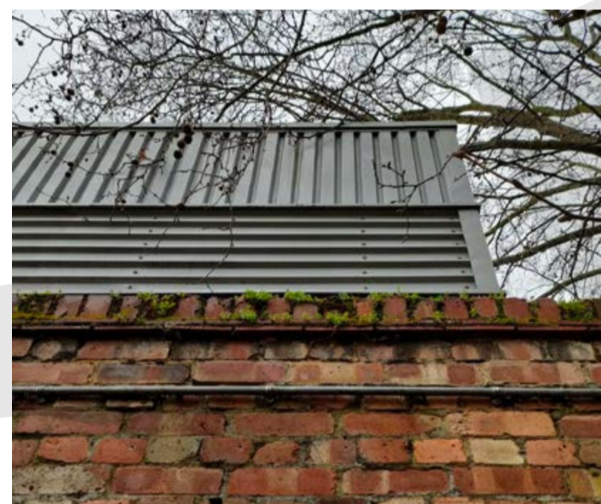
Brick and metal as the predominant materials
