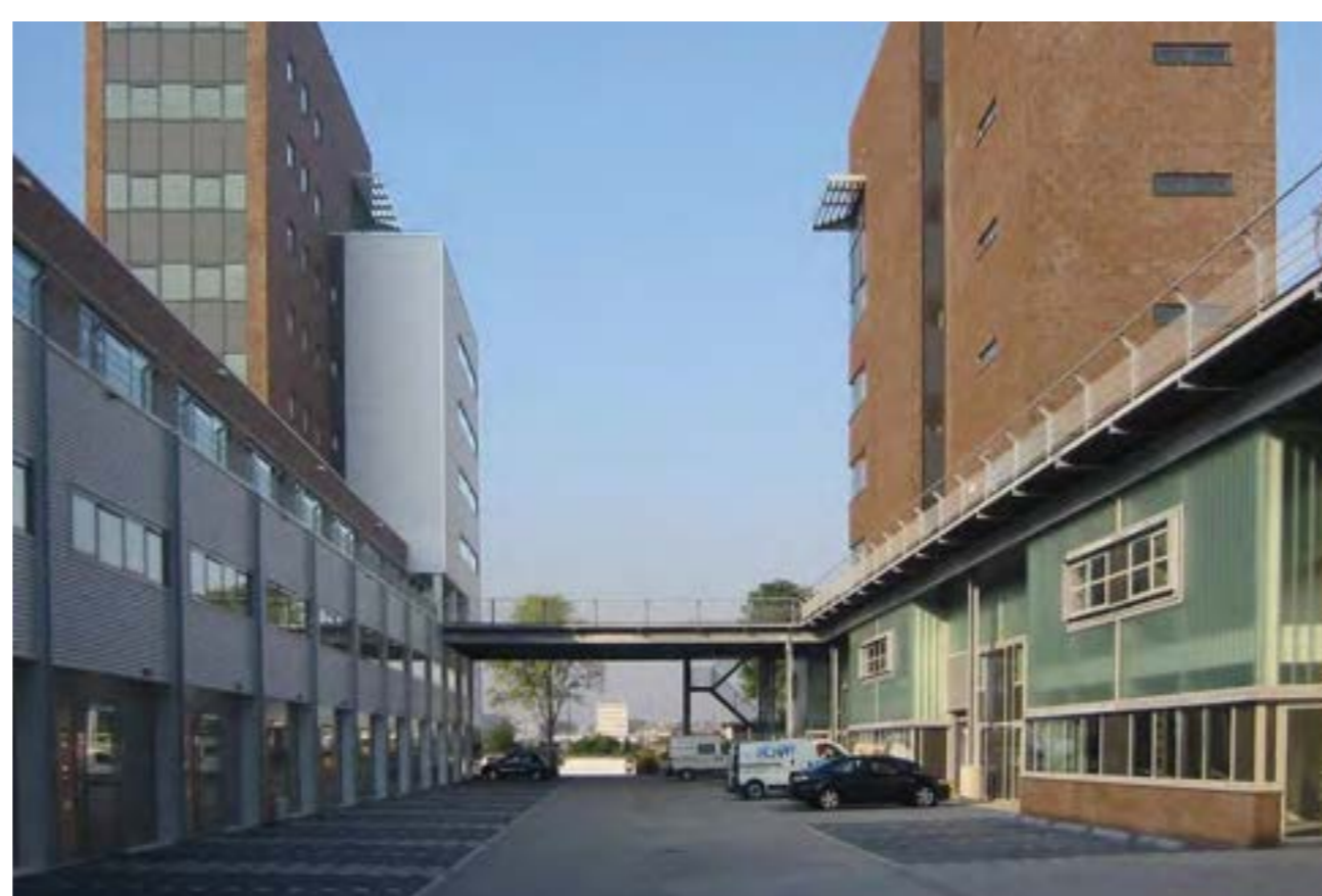
Kaap Noord, Amsterdam Medium-sized light industrial units are arranged around a central, shared service yard minimising the impact of yard-based activities on the surrounding area.
