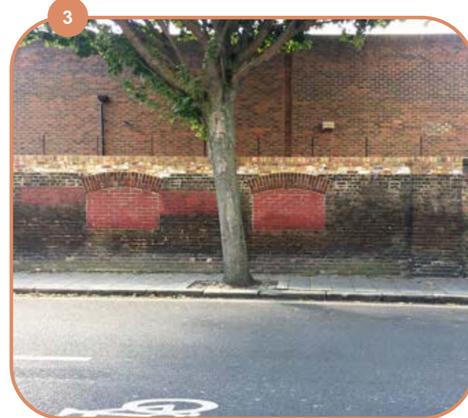
Remnants of the brick wall of Bricklayers Arms depot
