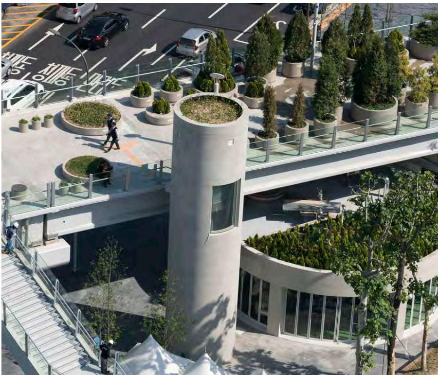
Planters and undercrofts
