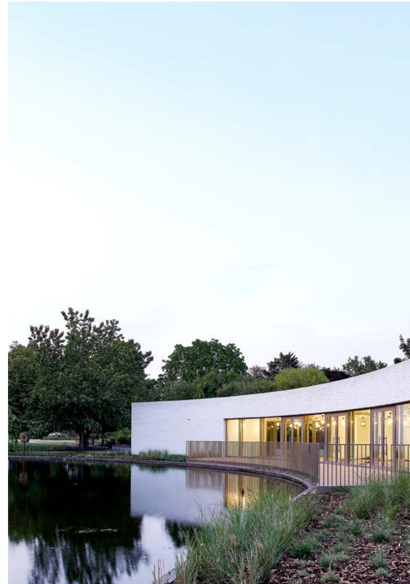
Southwark Park Pavilion, Bell Phillips Architects © Kilian O'Sullivan
